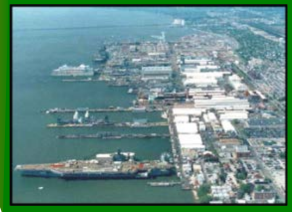
HII-NNS, VA Assembly, Test and Delivery
