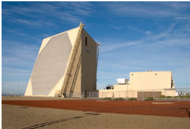
AN/FPS-132 Upgraded Early Warning Radar
